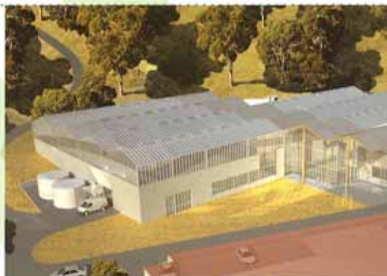
The Plant Accelerator, University of Adelaide, Waite Campus
